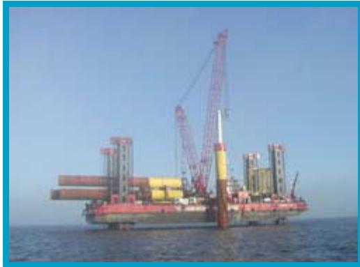
Plate 2.11 Monopile Hammer installation
