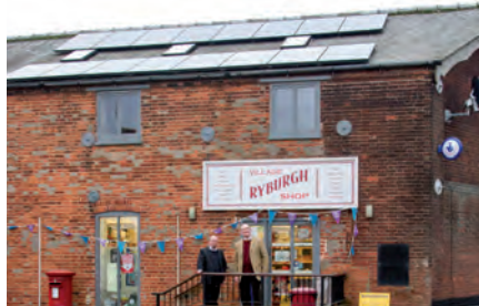
The Sheringham Shoal Community Fund funded solar panels for Great Ryburgh Village Shop
